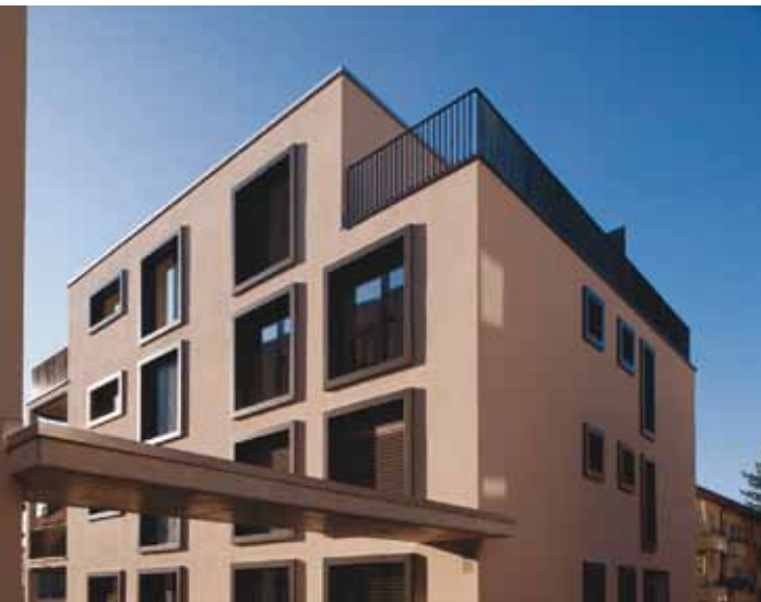
MFH, Bachhofnerstrasse, Zürich
